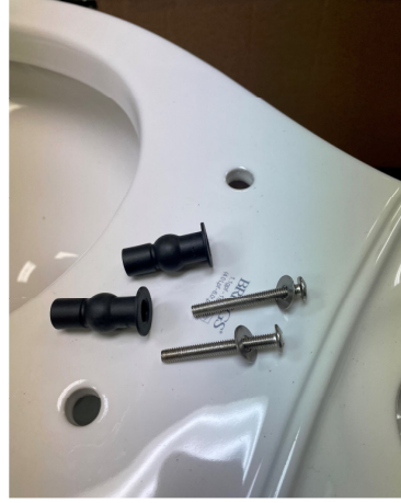
Separate the bolts and washers from the rubber grommets
