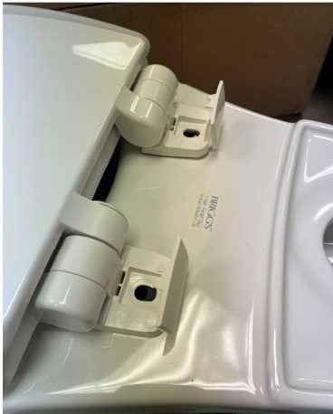
Take the bolt and insert it through the washer and seat hinge
