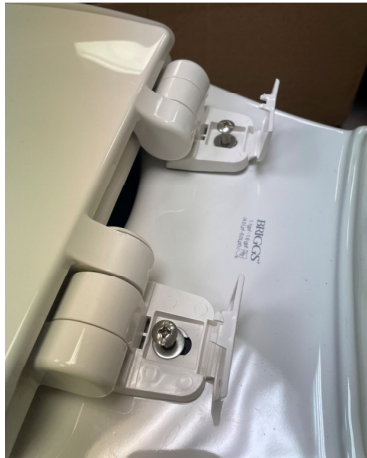
Insert bolts into the rubber grommets. Align the seat properly on the toilet bowl.
