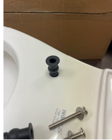
Insert rubber grommets into the toilet bowl holes
