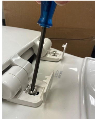
Screw down until the seat is tight
